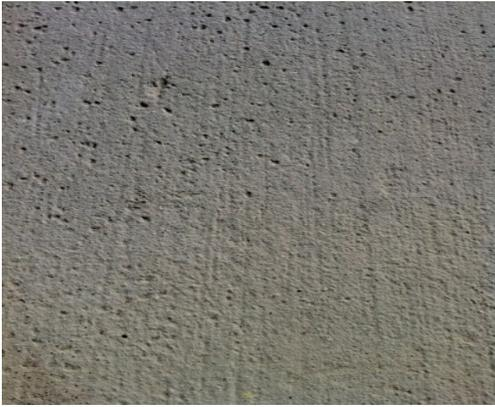
**Fig 4 Small Cavities in deck**
