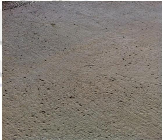
**Fig #2 Surface cavities in concrete**
