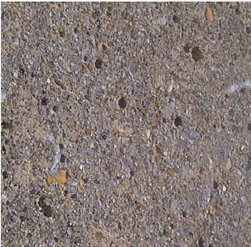
**Fig #1 Pinholes in concrete**
